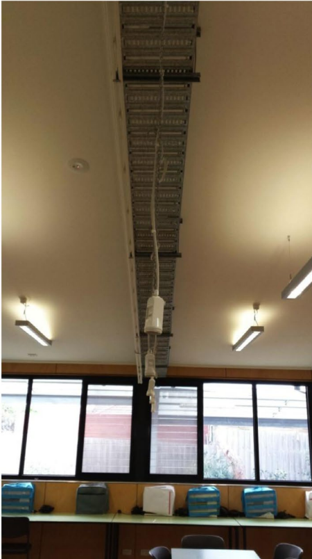
Figure 6. Newly installed power sockets in refurbished classrooms. These are located in ceilings and under whiteboards, meaning that they can only be used in full sight of a teacher (Lakeside).
